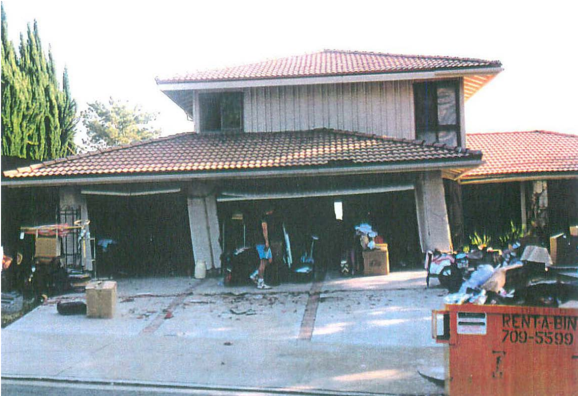
Major structure damage; heavy roof with inadequate sheer wall
