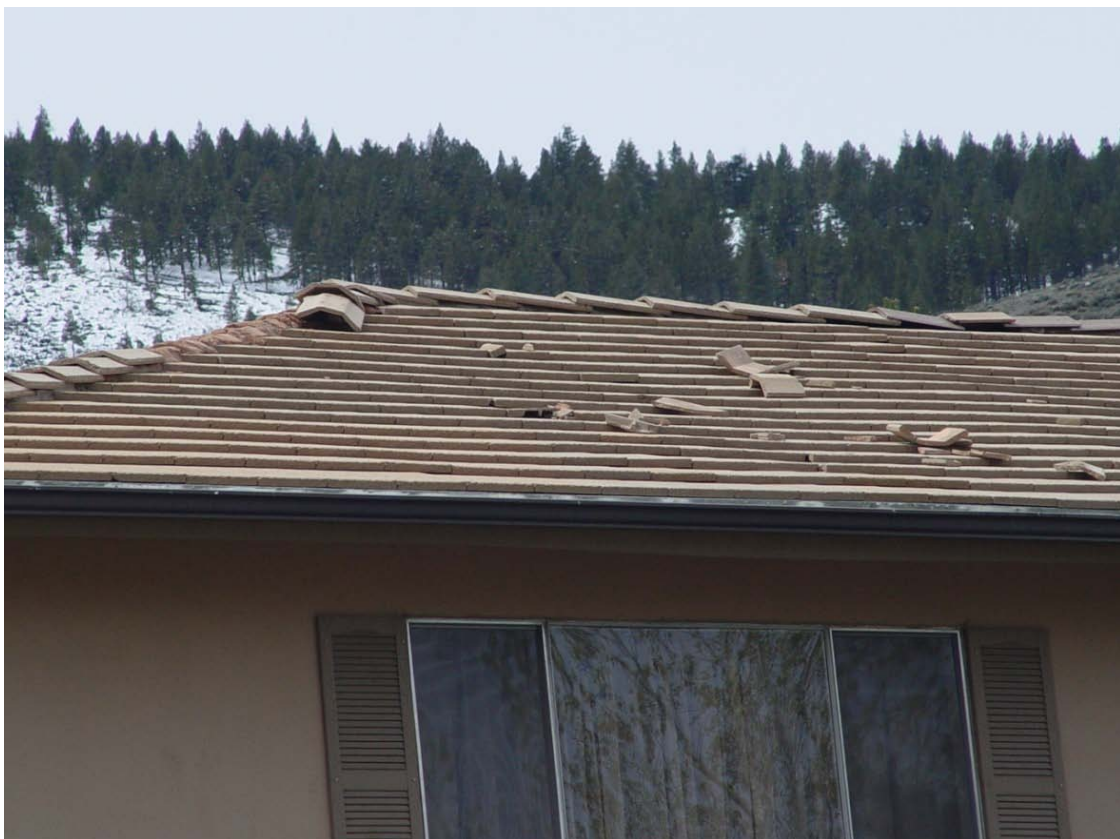
Wind damaged concrete shake
