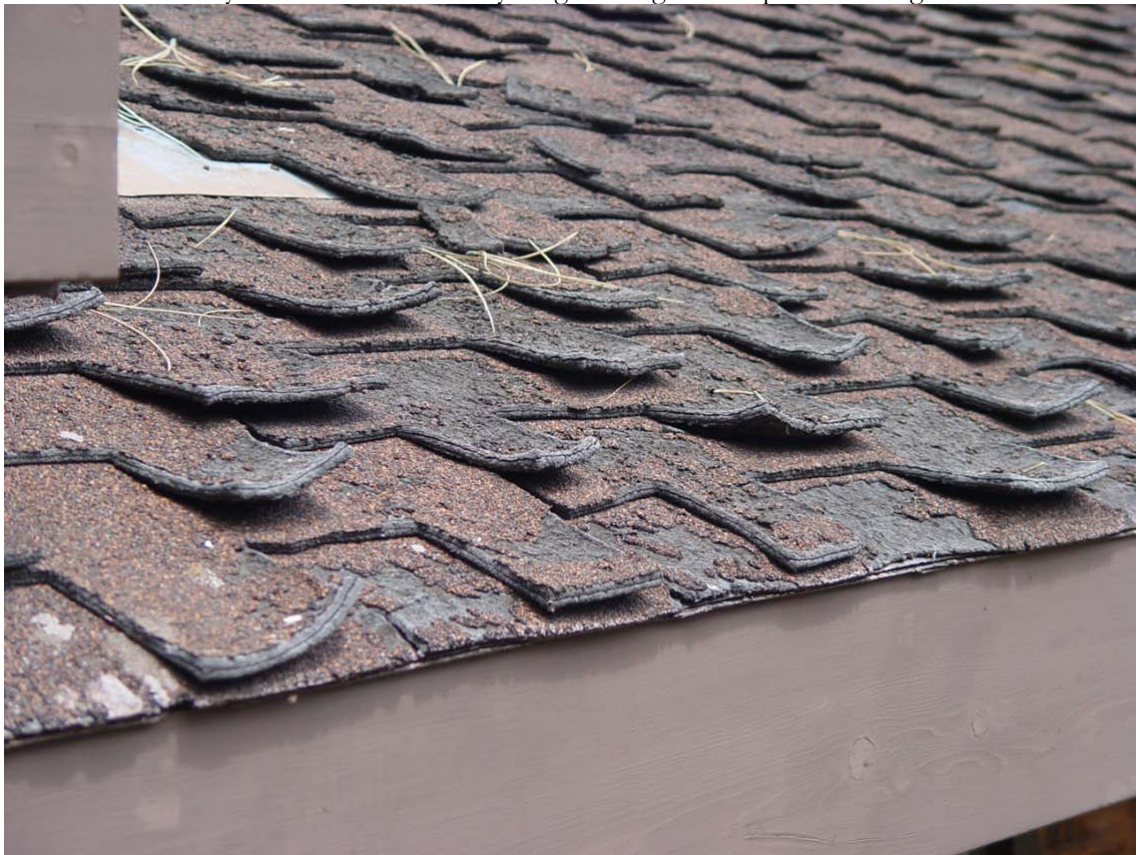
17-year old "50 Year" heavy weight fiberglass shingles
