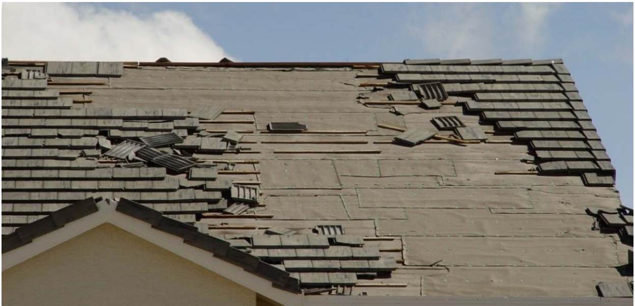
Wind damaged concrete shake
