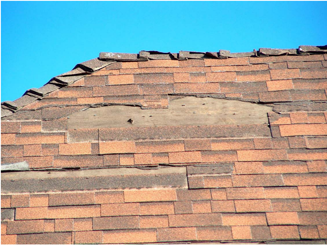
8-year old "30 Year" architectural fiberglass shingles
