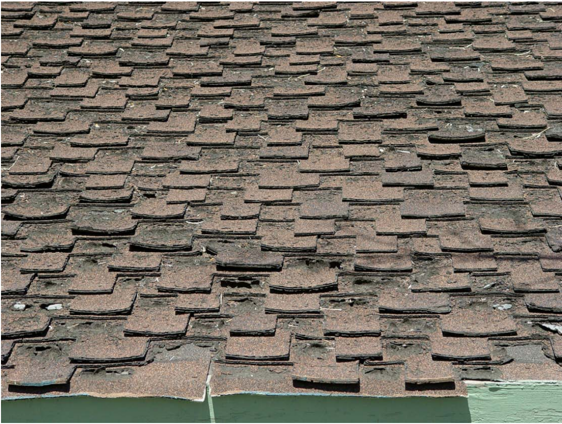
19-year old "40 Year" heavy weight fiberglass composition shingles
