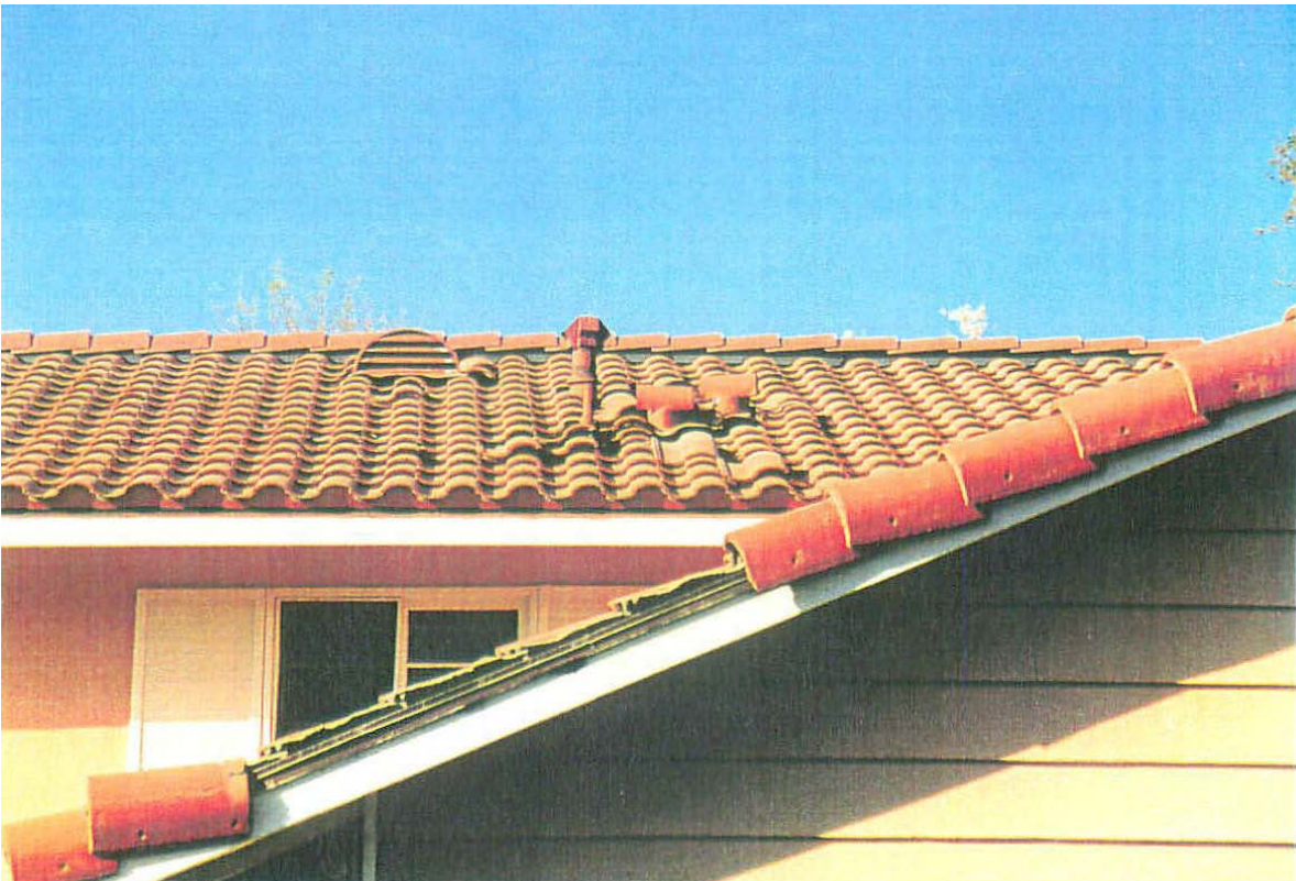
Displaced concrete tile, inadequate fastening
