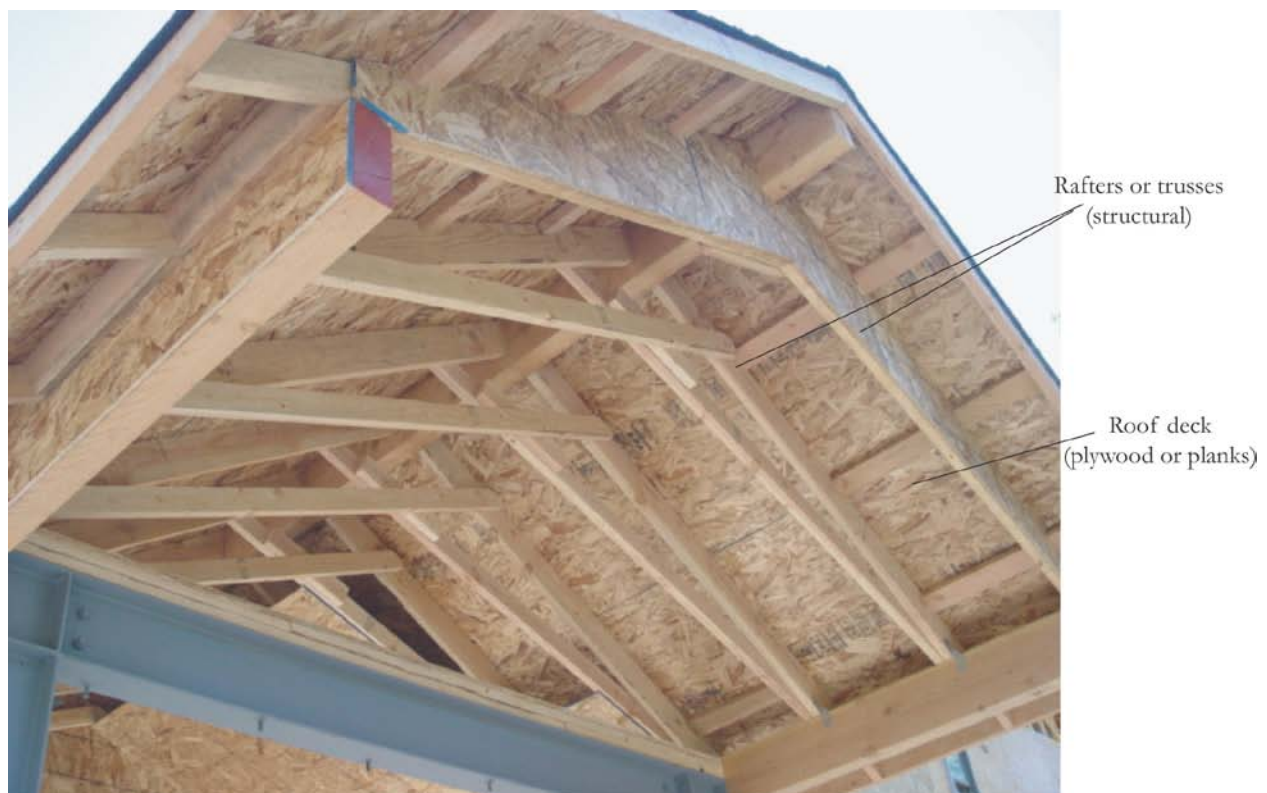
Diagram 2: Typical Sloped Roof Construction (What's Under the Roof Covering)
