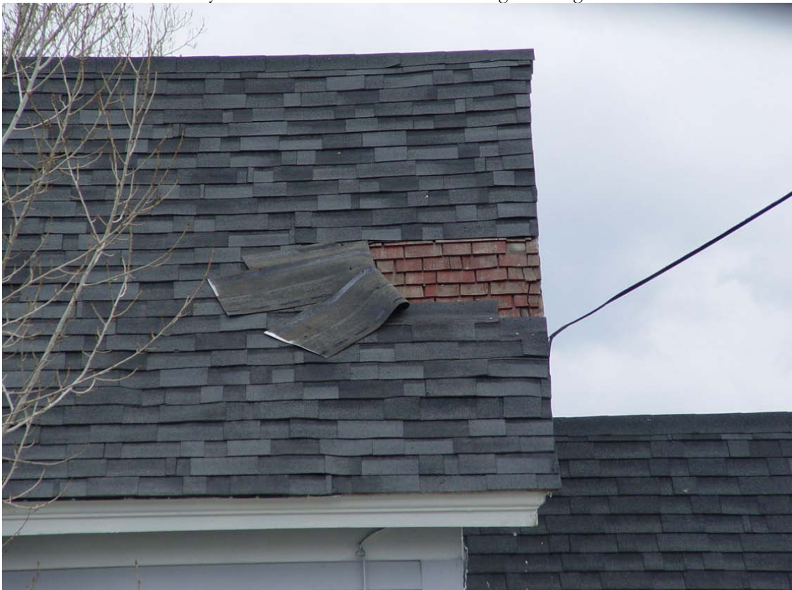
6-year old "30 Year" fiberglass shingles over wood shingles
