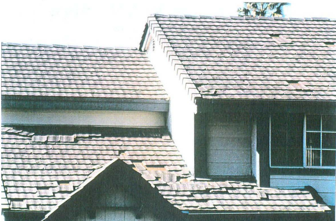
Inadequate fastening; concrete tile slipped
