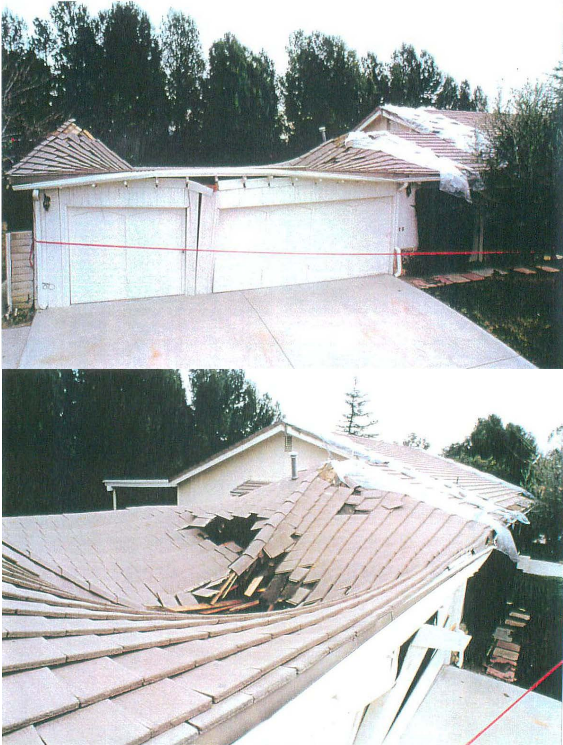
Concrete tile on 1"x6" skip sheathing, collapsed roof structure
