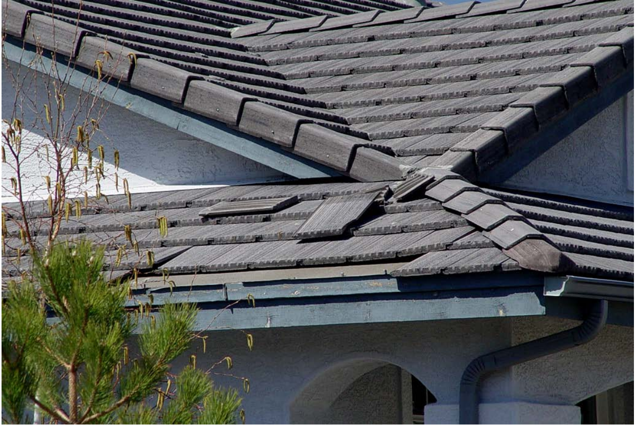
Wind damaged concrete shake
