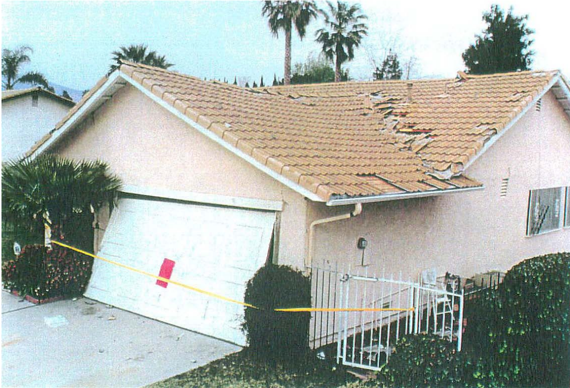
Concrete tile on 1"x6" skip sheeting; serious roof structure damage
